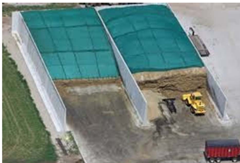
Figure 2. Storage of maize silage at the biogas plant location (concrete bunker silo with impermeable base and walls)
