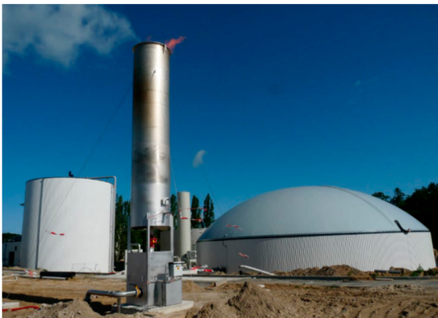
Figure 1. Biogas flare. (Source: Direct industry 1 )
