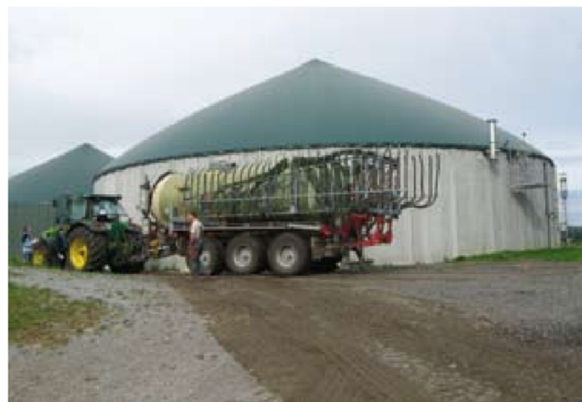
Figure 2. Digestate storage - covered to capture additionally released biogas. (Source: IEA Bioenergy 2 )
