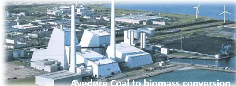
Avedøre Coal to biomass conversion
