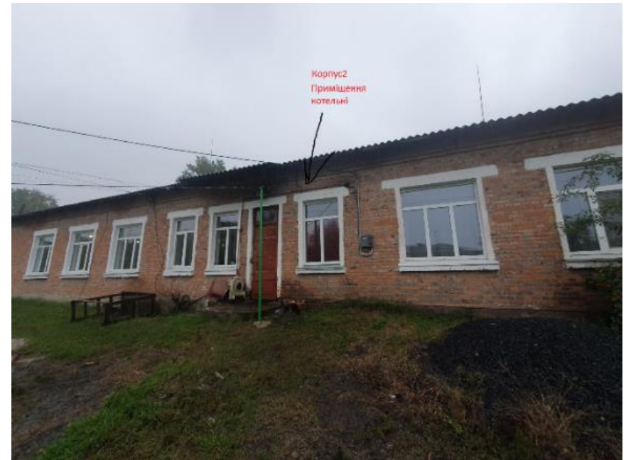
Image 2 Building 2, former boiler house facilities
